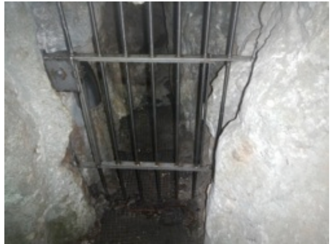
Physical controls on cave access are a tool for promoting compliance with cave access policy, where this cannot be achieved by other measures. Unfortunately, cave gates do not always guarantee compliance. This stainless steel gate replaces a mild steel gate which was damaged during a break-in at Kubla Khan Cave, Mole Creek Karst National Park, in 2009.
